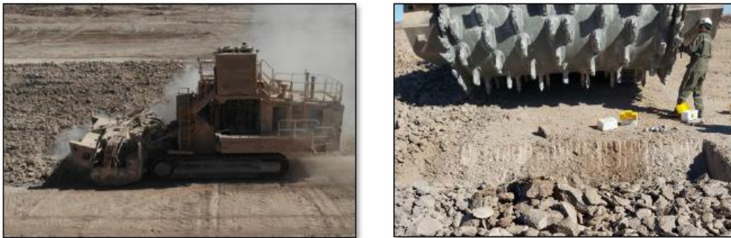
Figure 13-3. Terrain Leveler Surface Excavation Machine (SEM)
