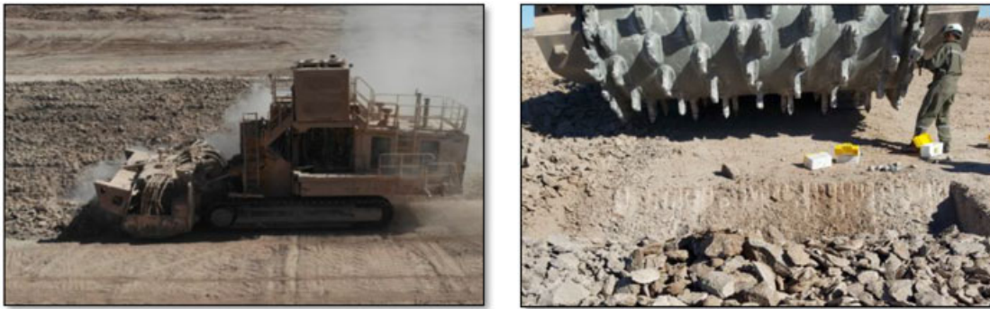
Figure 13-6. Terrain Leveler and SME equipment (Vermeer)
