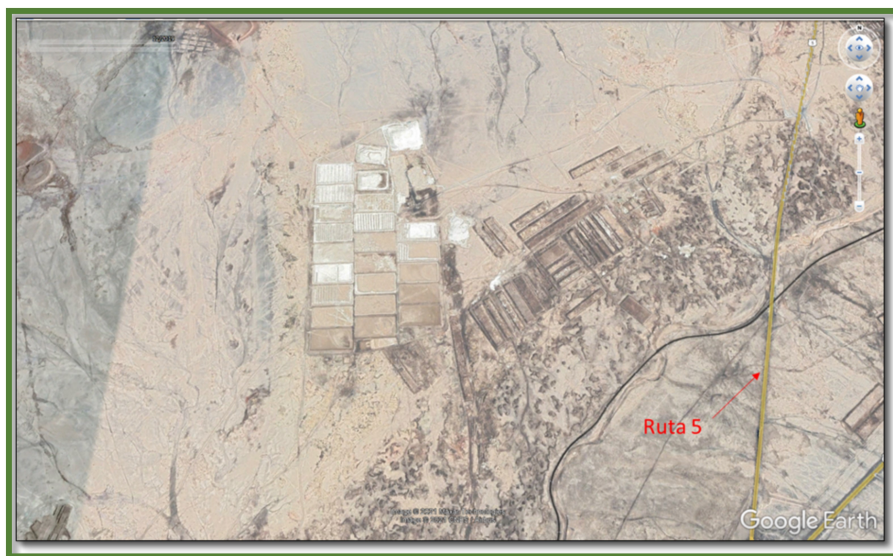
Figure 15-2. Status of the Plant Pampa Blanca
