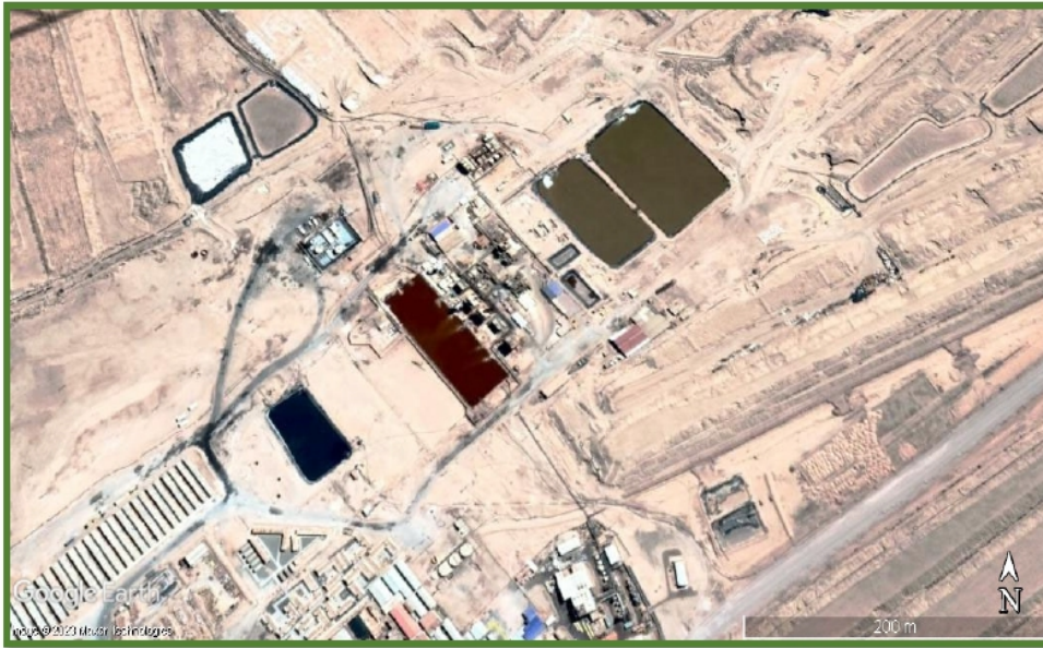
Figure 15-8. General View of The Iris Iodine Plant Area
