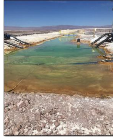
b) General view - production brine well and HDPE pipe for directing brine to the homogenization ponds
