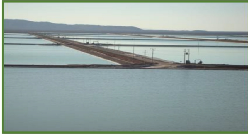
Figure 15-7. General View of Solar Evaporation Ponds in Sur Viejo
