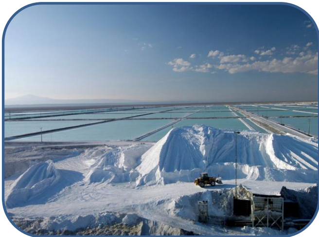
Photo: Evaporation ponds and silvinitic stock pile, Salar de Atacama
