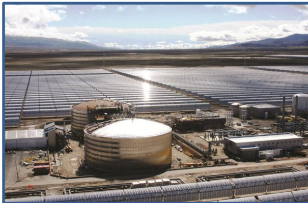
Photo: Andasol Millenium Power Station, Spain
